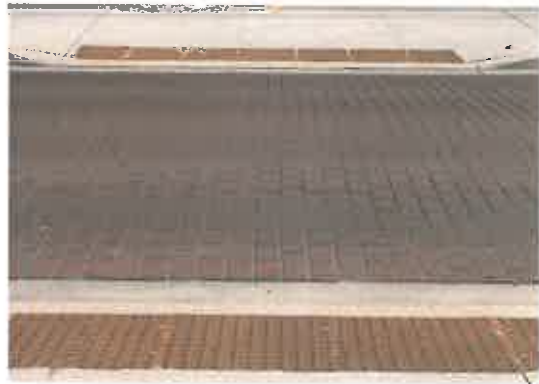
Figure 2.3: Pedestrian crossings should be designed to enhance visibility and calm traffic – Toronto, Ontario.
