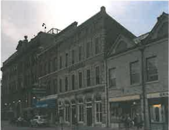
Figure 4.0: Repairing architectural features on existing buildings are encouraged – Kingston, Ontario.
