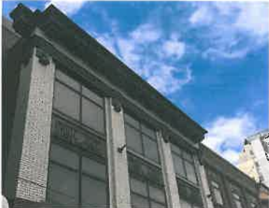
Figure 4.1: Maintaining architectural features on existing buildings are encouraged – Ottawa, Ontario.
