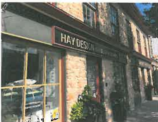
Figure 6.2: Embossed lettering set on architectural elements enhances a buildings' architecture – Perth, Ontario.
