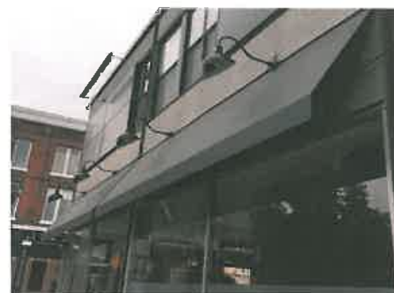
Figure 6.3: Signage awnings displaying business names with overhang lighting is encouraged – Pembroke, Ontario.
